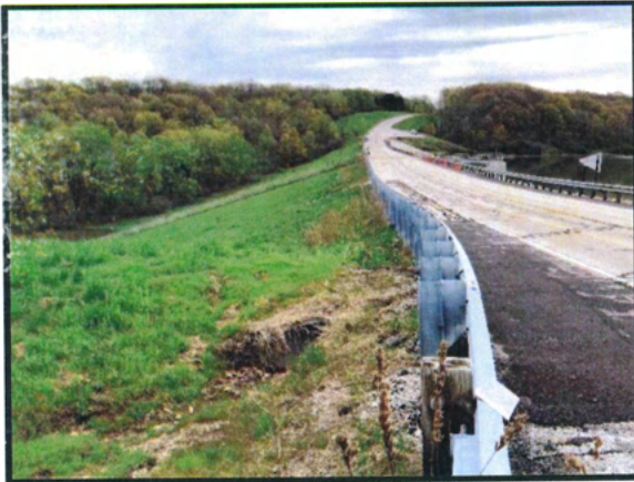
Fig. 21: Downstream face looking east
