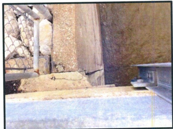
Fig. 12: Spillway wall at southeast corner of bridge
