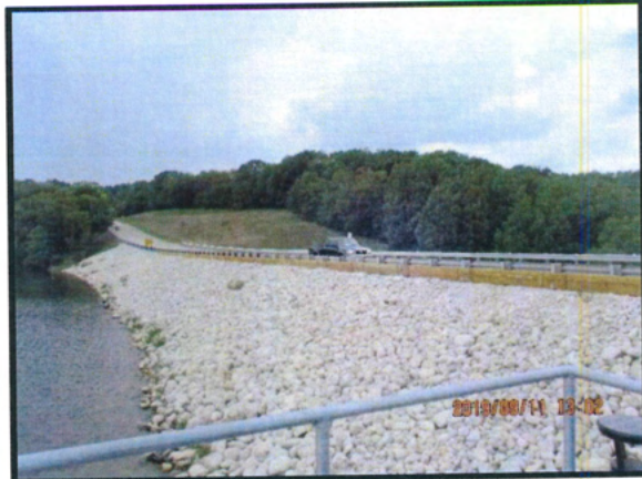
Fig. 52: West wave runup wall (Taken 09/11/2019)
