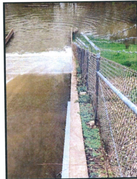
Fig. 34: East spillway wall and chute
