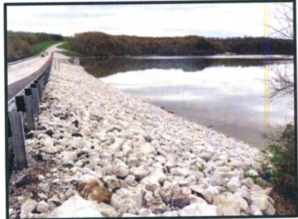
Fig. 18: Upstream face looking east
