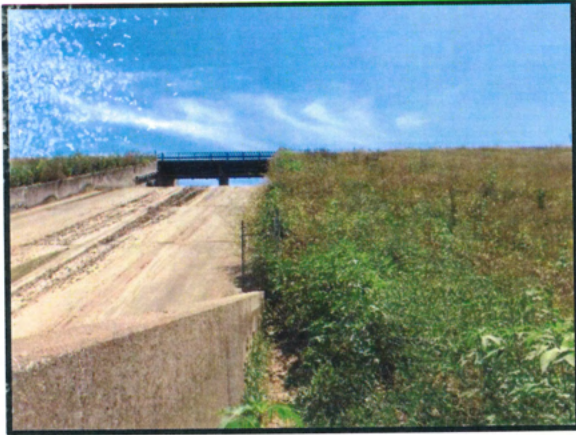
Fig. 51: West fence looking south (Taken 08/01/2019)
