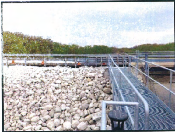
Fig. 09: Dewatering structure access walkway
