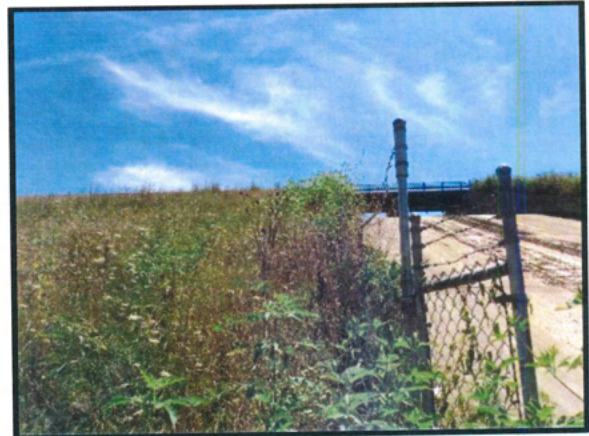
Fig. 42: East fence looking south (Taken 08/01/2019)
