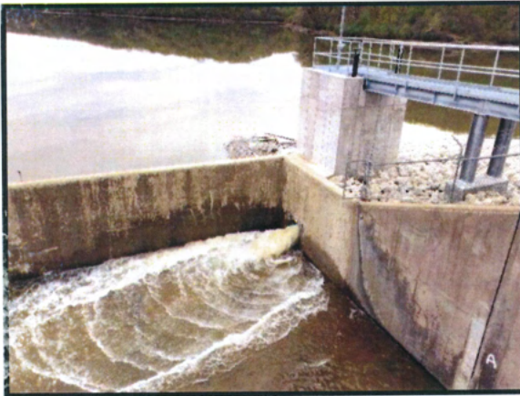
Fig. 05: Dewatering structure installed on west side of primary spillway
