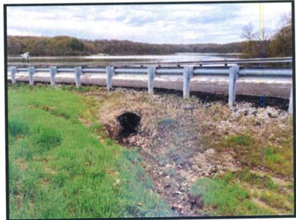
Fig. 20: West roadway RCP
