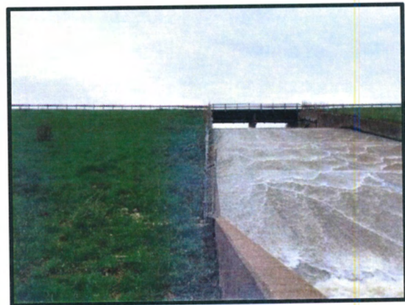
Fig. 38: Spillway fence looking south
