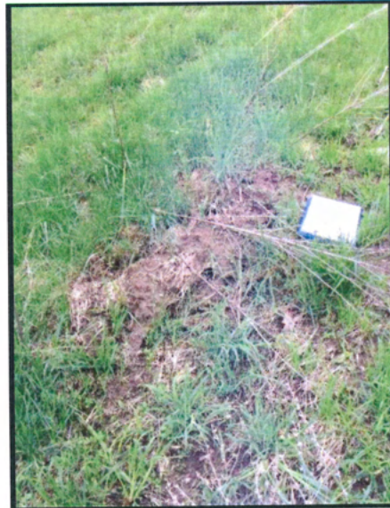
Fig. 36: Observed rutting east of spillway
