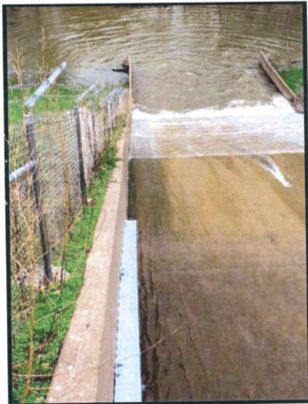
Fig. 33: West spillway wall and chute
