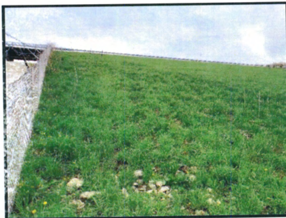
Fig. 29: Downstream face west of spillway
