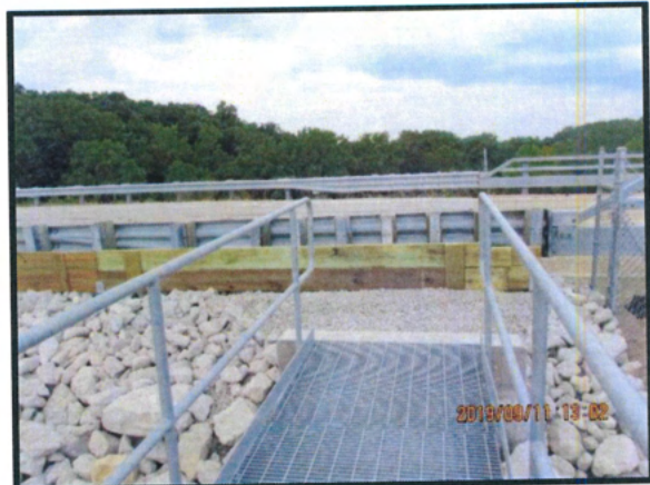
Fig. 54: West wave runup wall (Taken 09/11/2019)
