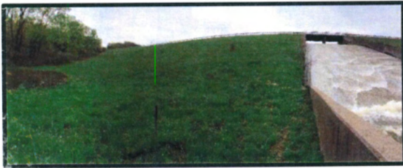
Fig. 35: Downstream face east of spillway
