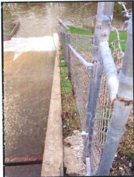
Fig. 15: Spillway wall at northeast corner of bridge
