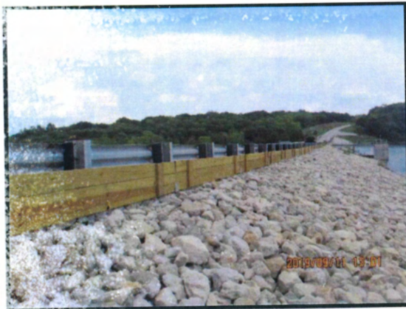
Fig. 55: West wave runup wall (Taken 09/11/2019)
