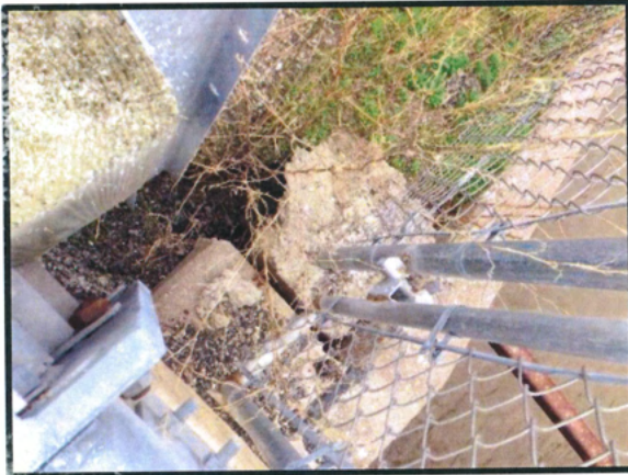
Fig. 13: Spillway wall at northwest corner of bridge
