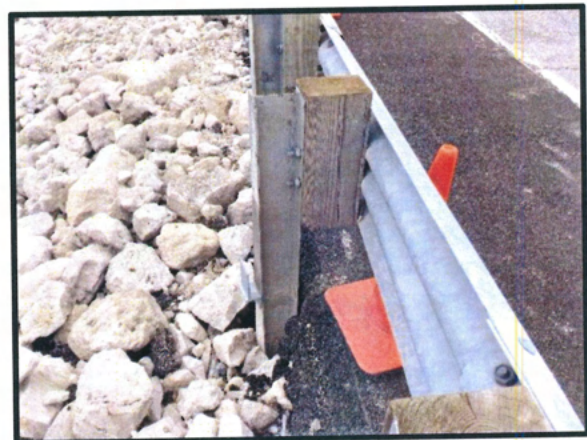
Fig. 16: HMA shoulder and brackets for wave runup wall installed 2018
