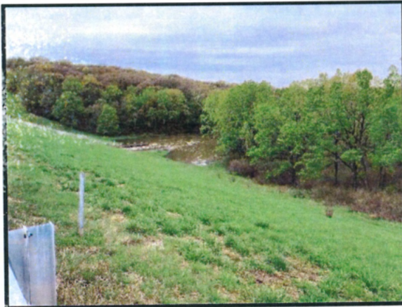
Fig. 03: Downstream dam face looking west
