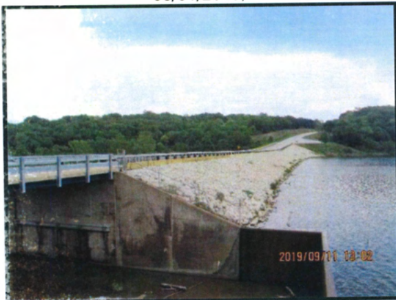
Fig. 53: East wave runup wall (Taken 09/11/2019)
