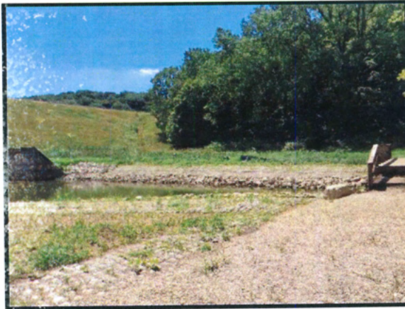
Fig. 41: Dissipater armored with riprap and cleared of vegetation (Taken 08/01/2019)
