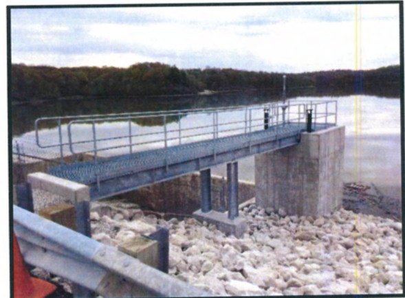
Fig. 04: Dewatering structure installed on west side of primary spillway
