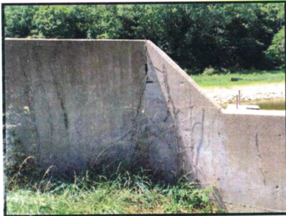
Fig. 45: East stilling basin wall (Taken 08/01/2019)
