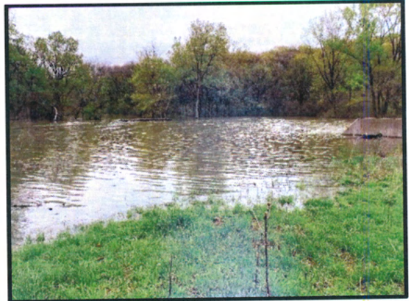
Fig. 26: Stilling basin and dissipater unable to be inspected 5/03/2019 due to flooding
