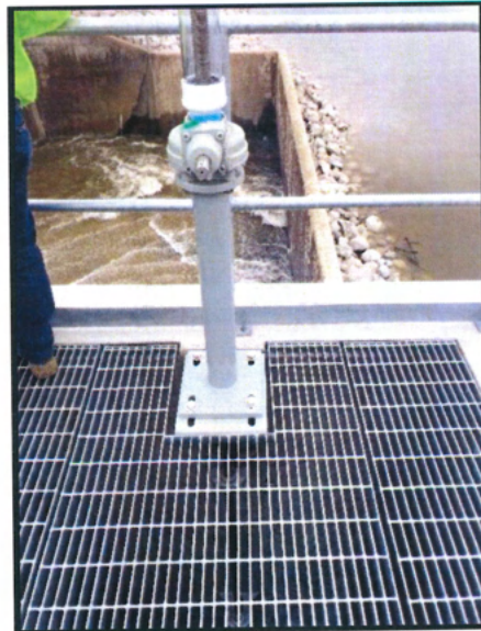
Fig. 10: Dewatering structure installed on west side of primary spillway
