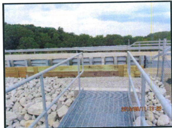
Fig. 56: West wave runup wall (Taken 09/11/2019)
