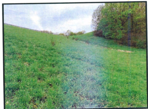
Fig. 30: Downstream face west of spillway
