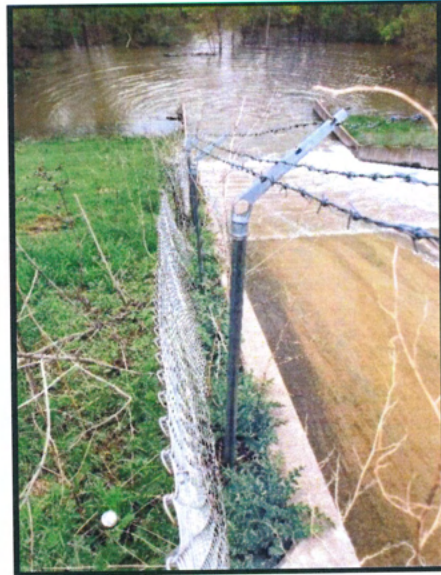
Fig. 32: West spillway fence
