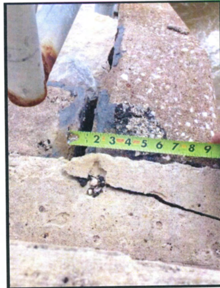
Fig. 14: Spillway wall at southeast corner of bridge
