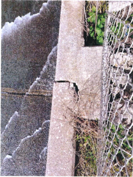
Figure 77: West spillway wall joint G
