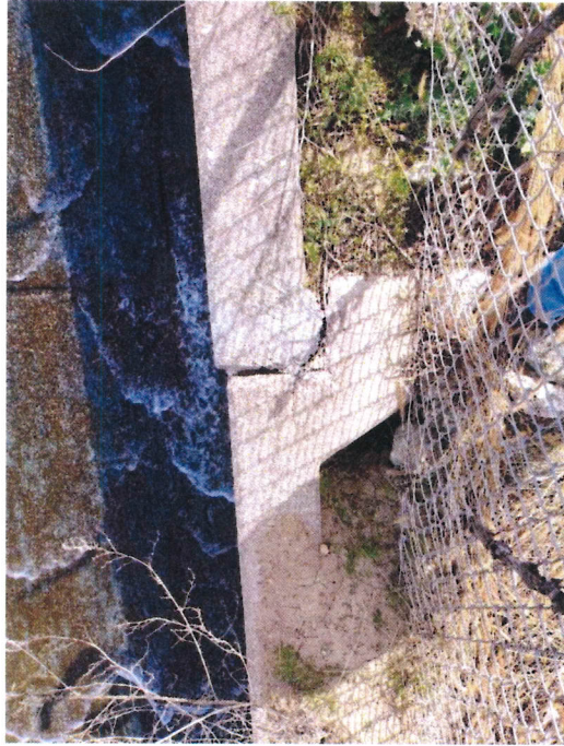
Figure 53: West spillway wall joint G
