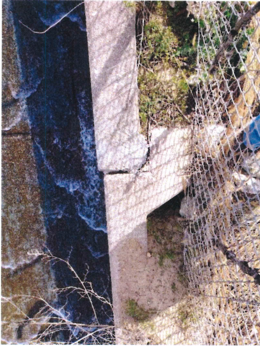
Figure 53: West spillway wall joint G
