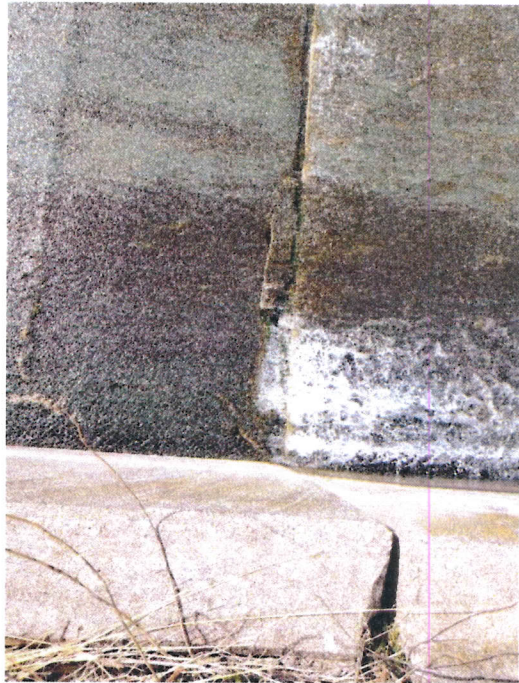
Figure 83: Chute slab spill joint E
