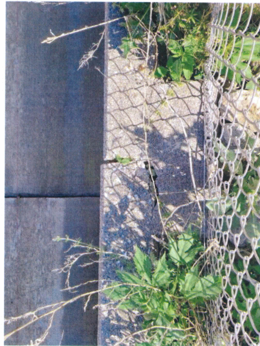
Figure 63: West spillway wall joint G
