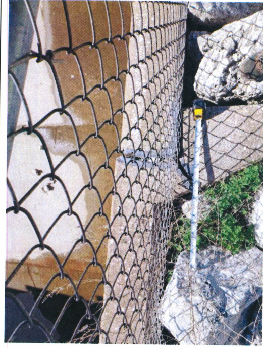
Figure 18: West spillway wall joint A
