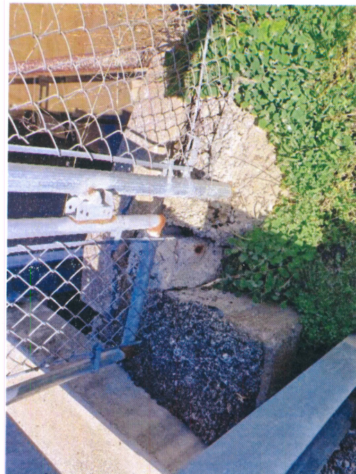
Figure 74: East spillway joint C
