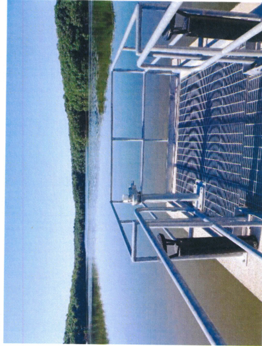
Figure 23: Sluice gate floor stand
