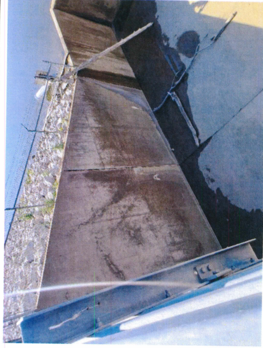
Figure 10: Southeast spillway wall looking southeast
