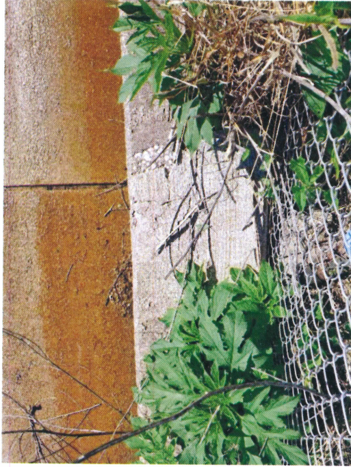
Figure 45: West spillway wall joint F
