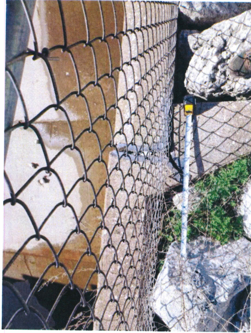
Figure 18: West spillway wall joint A
