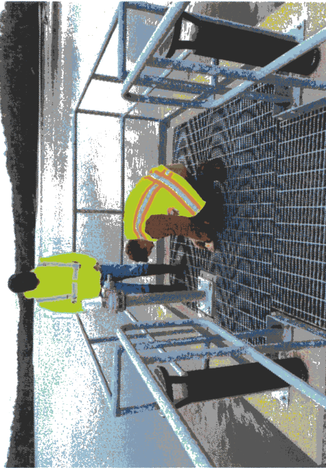
Figure 21: Sluice gate floor stand
