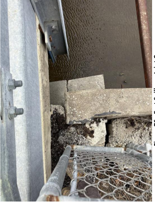
Figure 76: East Spillway Joint C
