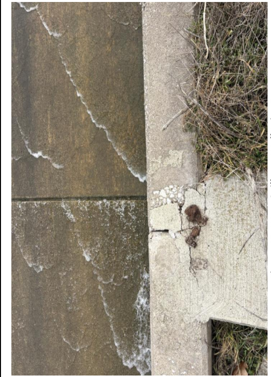
Figure 45: West Spillway Wall Joint F
