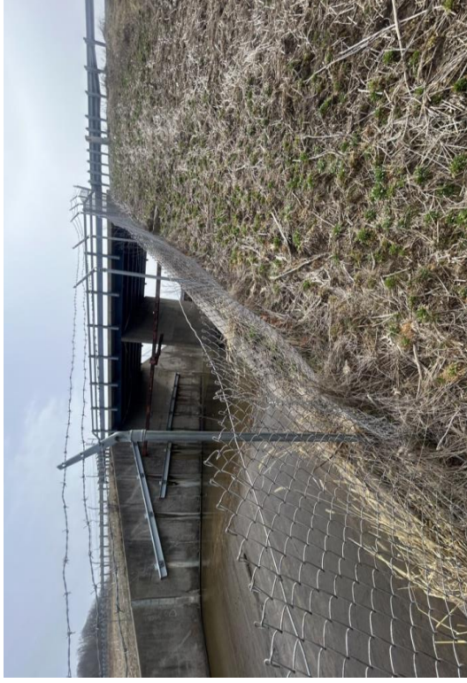
Figure 38: Fence Displacement
