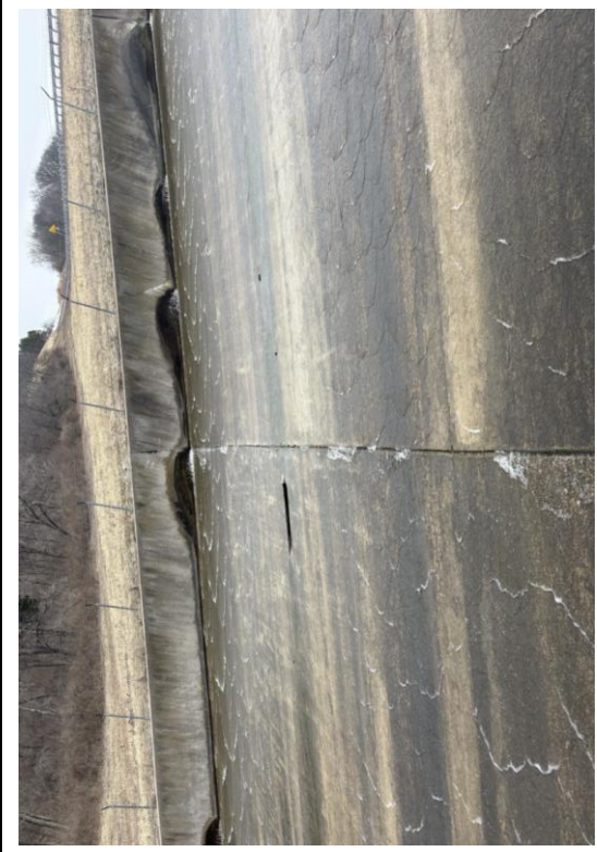
Figure 46: Spillway Floor Joint F, Looking East
