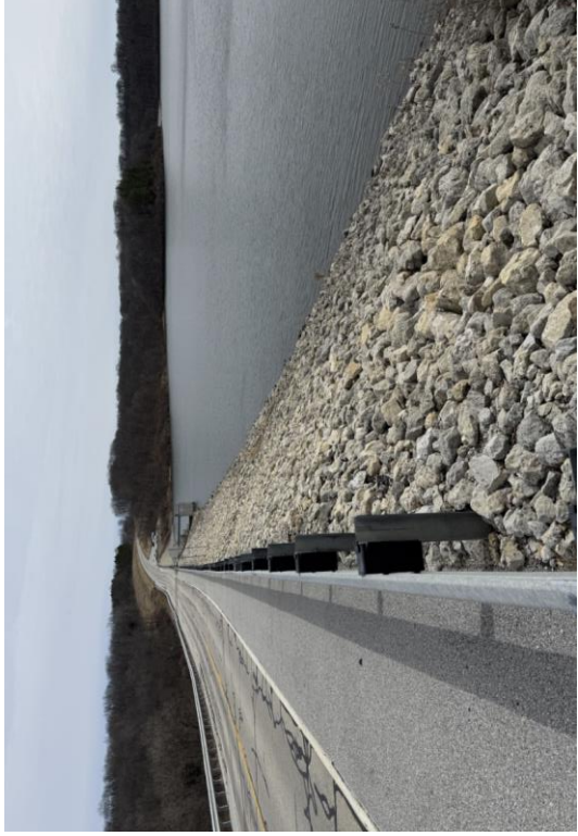
Figure 24: Upstream Slope Protection Looking East
