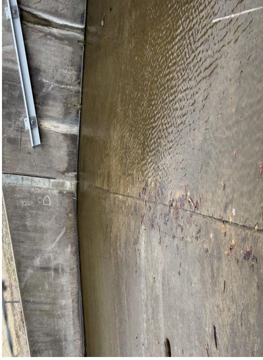
Figure 42: Spillway Floor Joint D, Looking East
