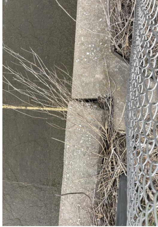
Figure 73: East Spillway Wall Joint E
