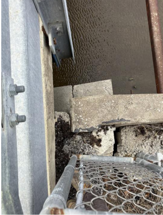
Figure 77: East Spillway Joint C
