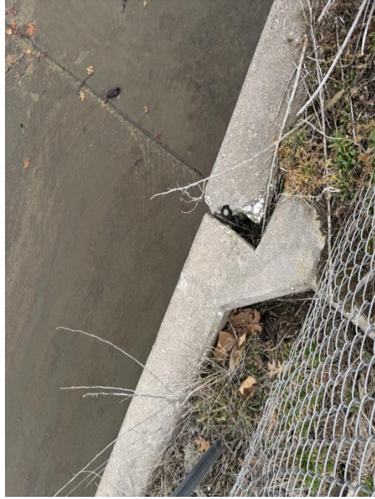
Figure 41: West Spillway Wall Joint D
