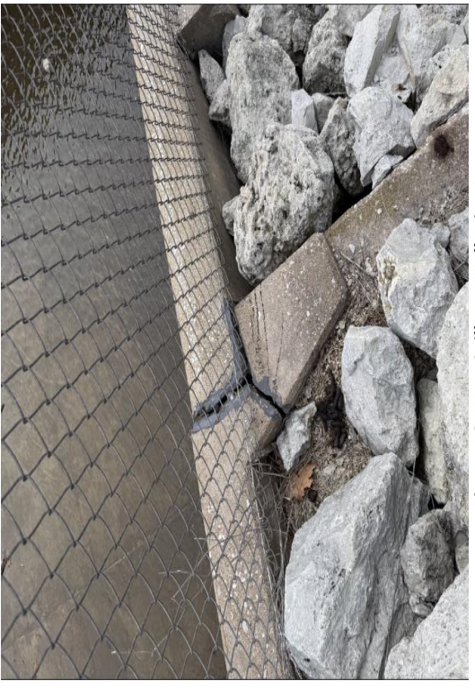
Figure 16: West Spillway Wall Joint A
