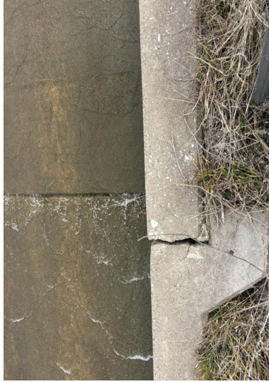
Figure 43: West Spillway Wall Joint E
