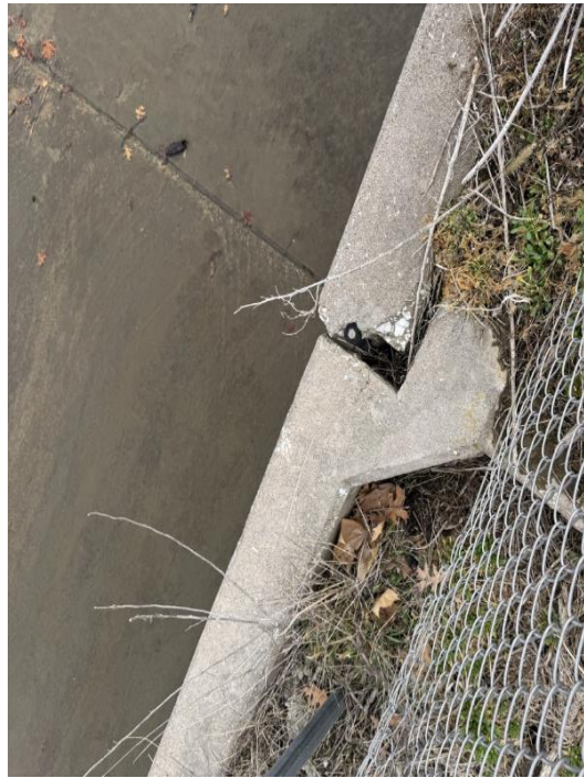
Figure 41: West Spillway Wall Joint D
