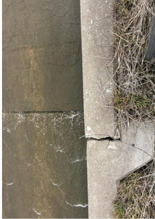
Figure 43: West Spillway Wall Joint E
