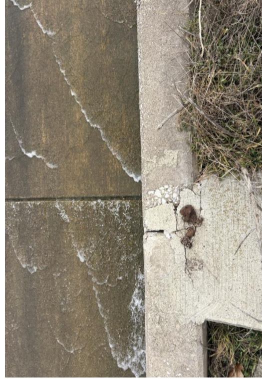
Figure 45: West Spillway Wall Joint F
