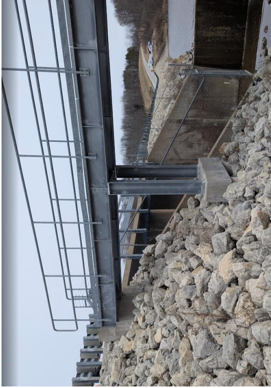
Figure 23: Ramp Substructure to Sluice Gate Outlet Structure
