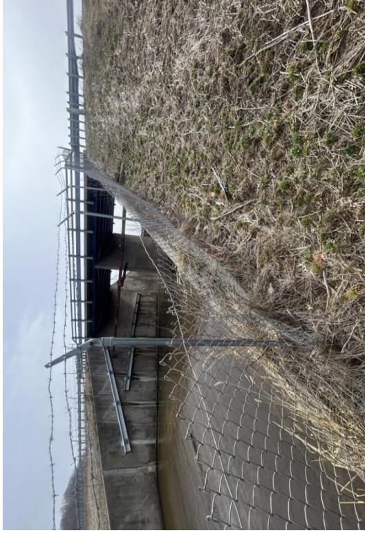
Figure 38: Fence Displacement
