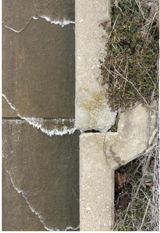
Figure 48: West Spillway Wall Joint G
