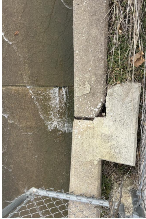
Figure 51: West Spillway Wall Joint H
