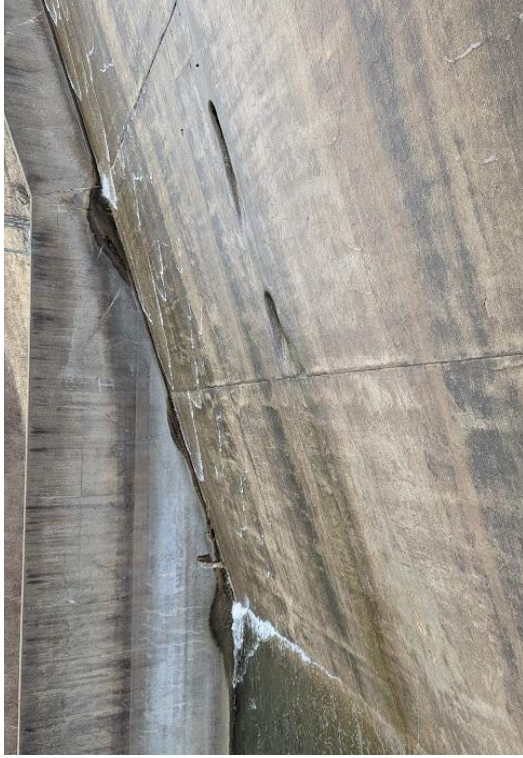
Figure 65: Spillway Floor Joint I, Looking East
