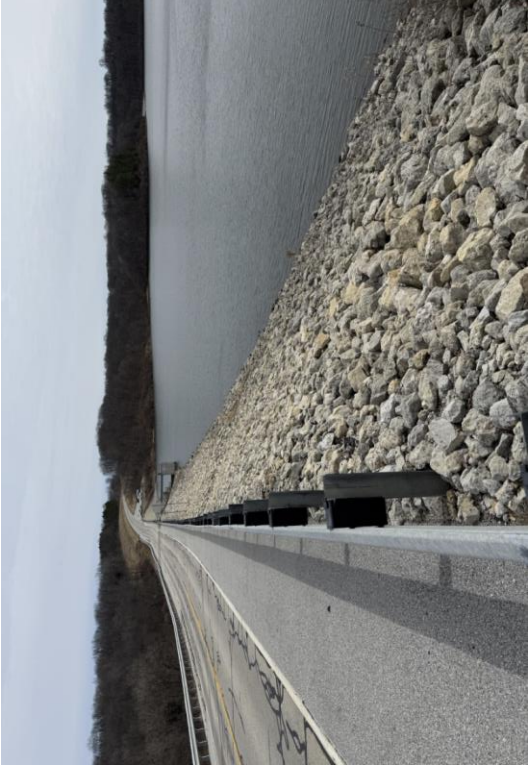
Figure 24: Upstream Slope Protection Looking East
