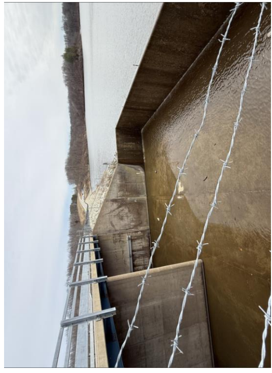
Figure 12: Southeast Spillway Wall Looking East
