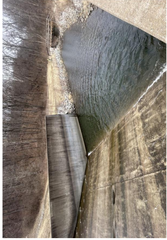
Figure 64: West Spillway Wall Elevation Looking Northwest
