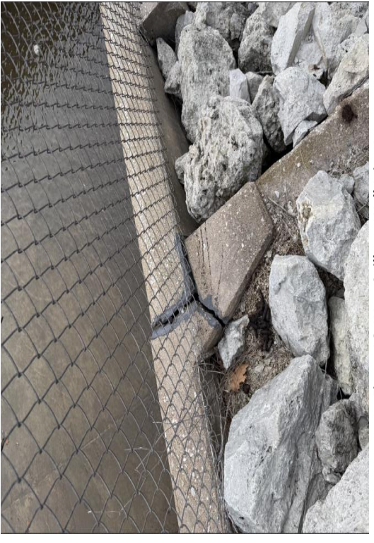
Figure 16: West Spillway Wall Joint A
