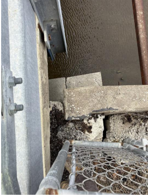
Figure 77: East Spillway Joint C
