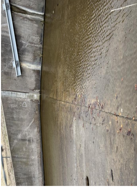
Figure 42: Spillway Floor Joint D, Looking East
